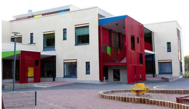
The Vanttila kindergarten, with multi-part infill panel windows.
