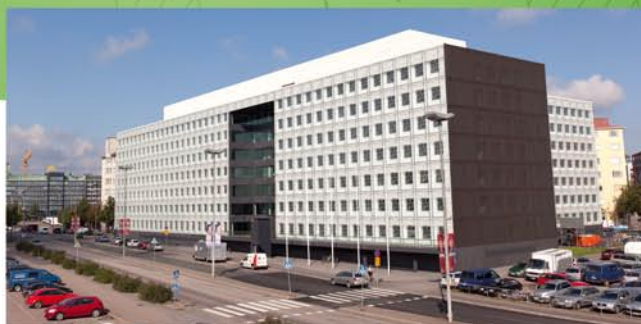
Hakaniemi, Helsinki – the Finnish National Board of Education building. In total, 760 windows equipped with solar protection glass and grey frames.
